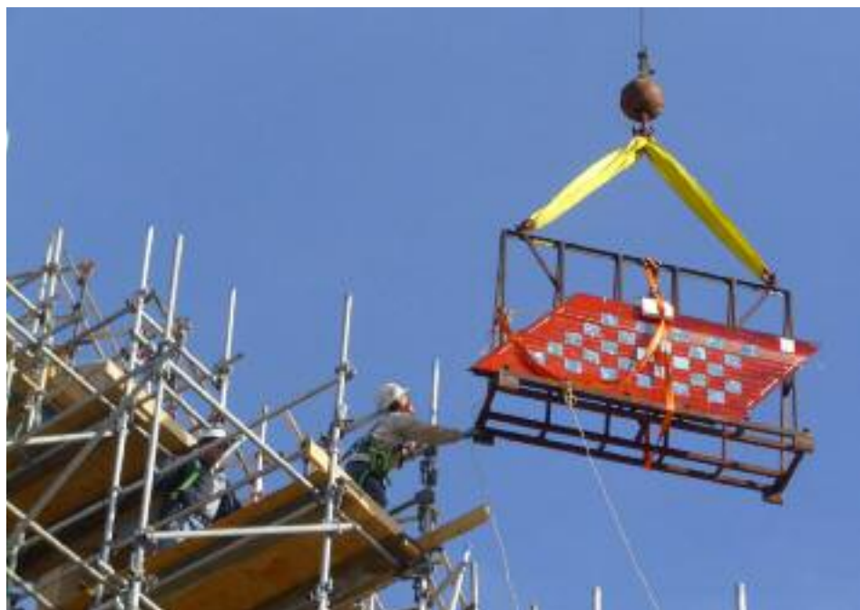
The solar stained glass panels were carefully installed in May 2011.
